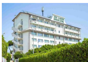
a. l'Over Aris Garden residence
